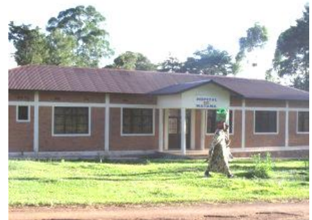
Administration block Matana hospital
