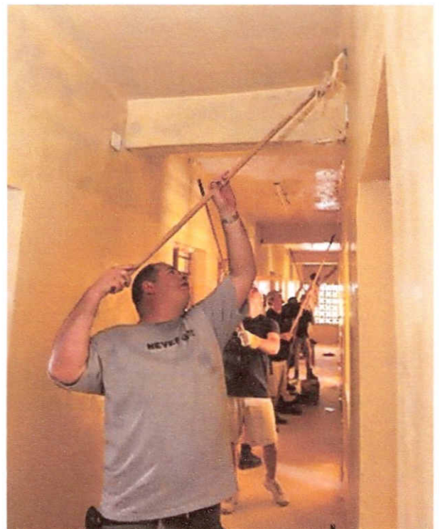
Members of the crew paint the walls at the shelter.
