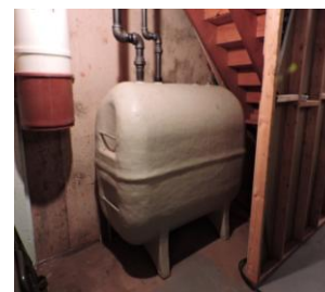
New fiberglass oil tank
